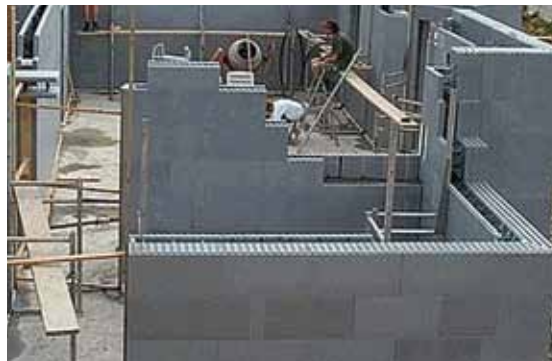
Insulating Concrete Forms (ICFs)
